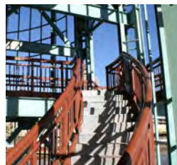
The Wabash Street Bridge in St. Paul, MN has a staircase that connects the bridge to a trail. The design of the staircase's structure also serves as a "gateway icon" on the bridge. A small plaza is located at the top and another at the bottom of the stair core.
