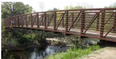
A simple design defers to the natural setting. Los Alamitos Creek Bridge - San Jose, CA
