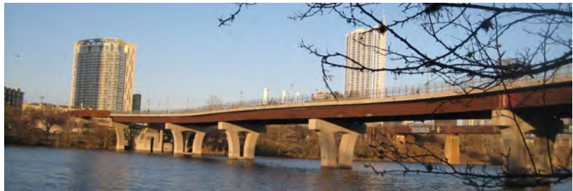
View of bridge piers and the city beyond.
