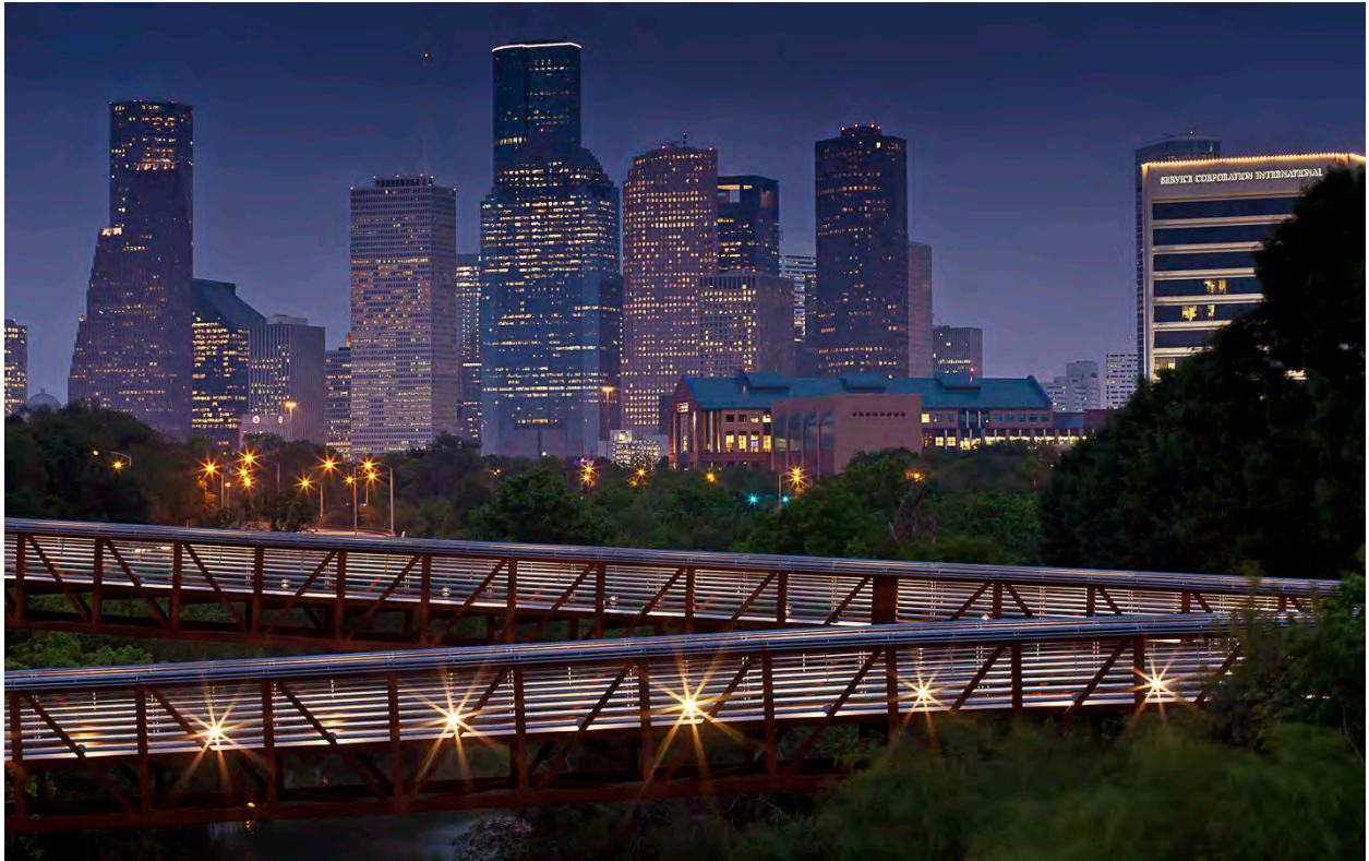
The Rosemont Bridge railings include hundreds of lights that illuminate the pathway at night and frame the view of downtown Houston's skyline.
