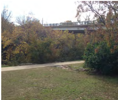
North San Gabriel River Trail at bridge.
