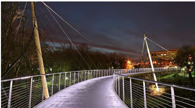
Nighttime view of bridge (photo credit: James Wellman)
