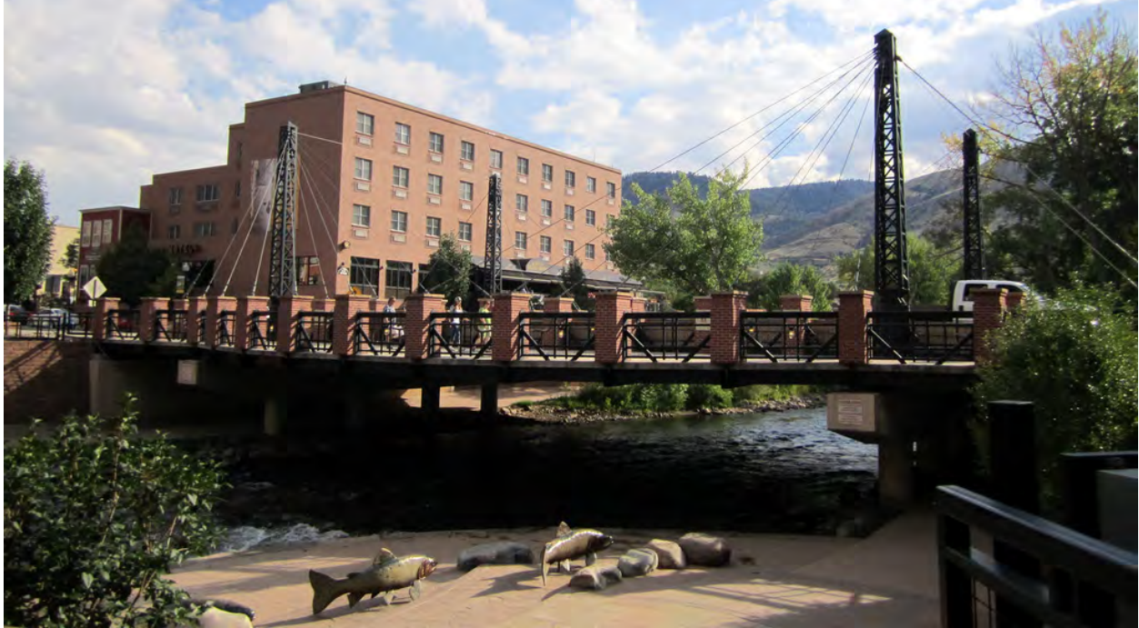
The bridge includes four towers holding up the pedestrian plazas with stay cables. Directly southeast the bridge are mixed use buildings with residents and offices overlooking the creek.
