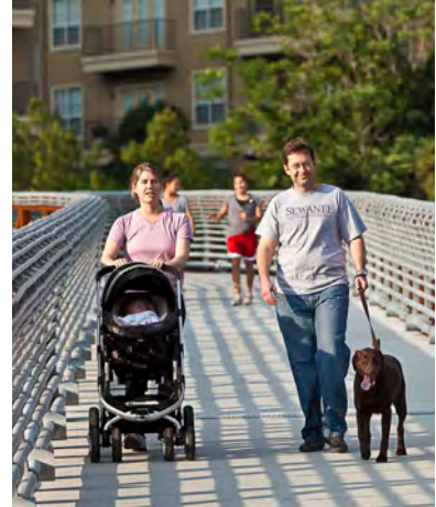
The bridge is accessible and safe for strollers.
