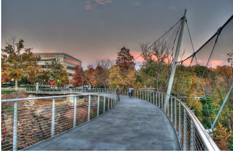
The bridge features lightweight metal railings and concrete floor. (photo credit: Crowefly images)
