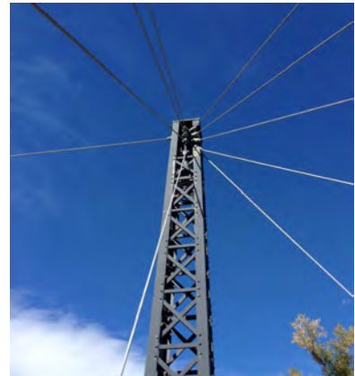
The fan design of the cables holds up the pedestrian plazas.
