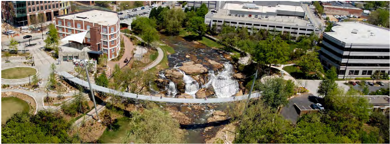
The bridge is suspended and arched away from the falls with two 90-foot masts. Plazas are provided on either side of the bridge.
