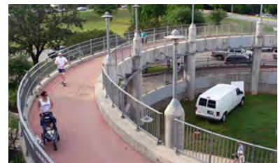
Ramps may be used to connect between the bridge and trails.
