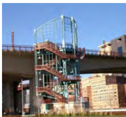
The Wabash Street Bridge in St. Paul, MN has a staircase that connects the bridge to a trail. The design of the staircase's structure also serves as a "gateway icon" on the bridge. A small plaza is located at the top and another at the bottom of the stair core.
