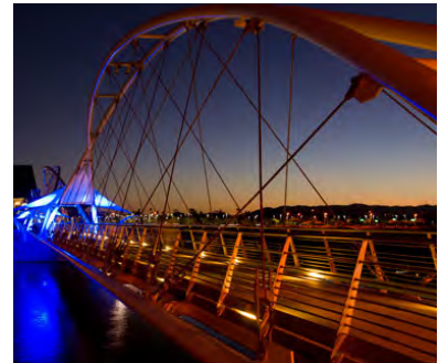
The pedestrian bridge at Tempe Town Lake in Tempe, AZ offers a unique experience at night with a whimsical colored lighting scheme.
