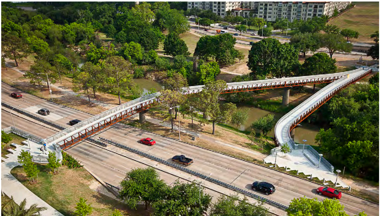
The bridge crosses Memorial Parkway and the bayou and then zig-zags back to the north bank of the bayou to link in with both sides' hike and bike trails. A small plaza is provided at each "landing".
