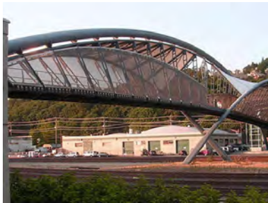
A distinctive design enhances tourism. Elliott Avenue Bridge - Seattle, WA
